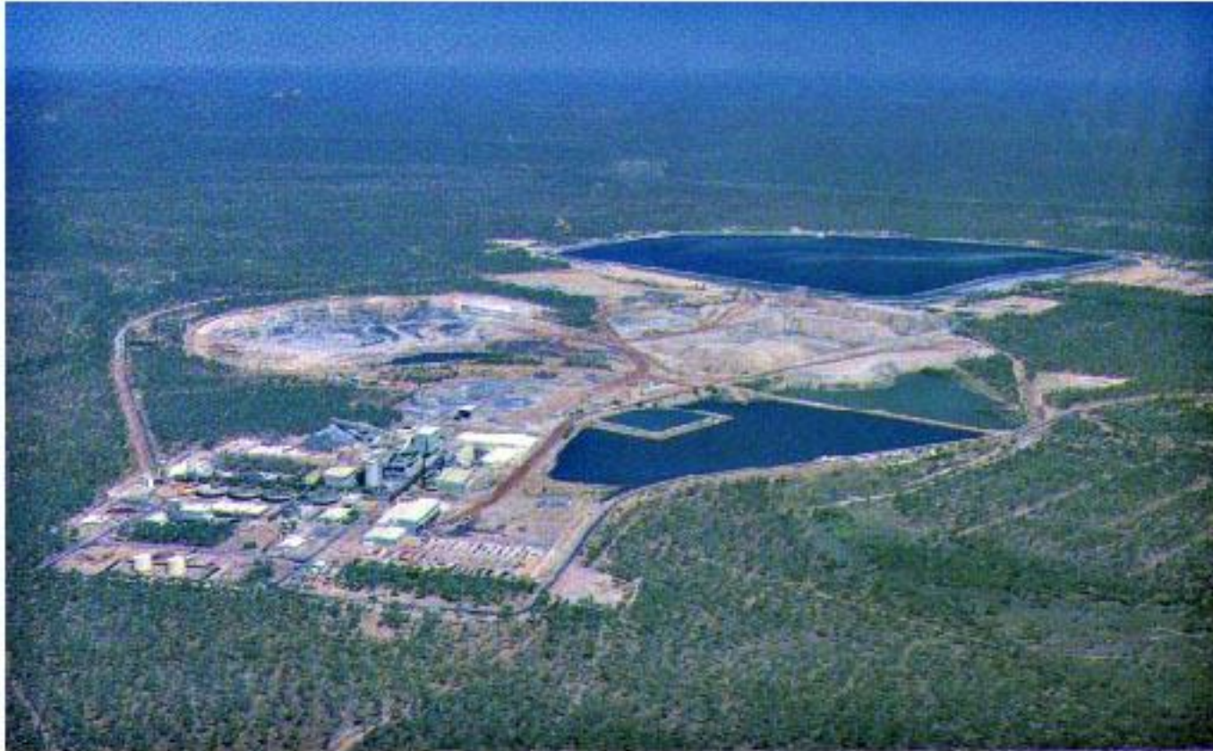
Aerial view of Ranger Mine and Plant
